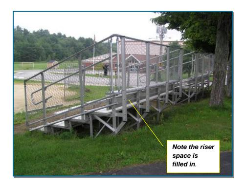
Close up of prior photo showing the riser protection, fencing and bottom rails.
