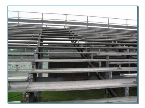
This is an older, permanent bleacher system at a high school football field. This system has been retrofitted to some degree. There is no riser fall protection and no hand rails in the aisle walkway. However, fencing has been added to the top and sides reducing the potential for falls from the bleachers. Riser gaps should be closed to reduce the potential for falls between the seat and walking surfaces, especially for children. The installation of aisle railings is recommended.
