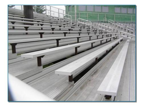
This photo shows a newer, permanent bleacher system at a town recreational baseball field. The system has aisle railings, riser protection, and top and side guardrails with mesh fencing. The risers should prevent falls between the seat-boards and the floorboards and should also prevent objects from falling from the floorboards onto anyone beneath the bleachers.
